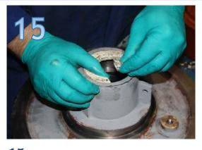
**15**. Install rope packing (Picture 15) in stuffing box.
